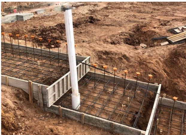
Storm Sewer installed Fitness Center
