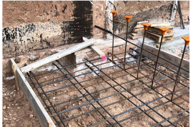
Footings and rebar installed Fitness Center
