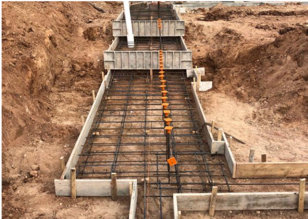
Step Footings and rebar installed Fitness
