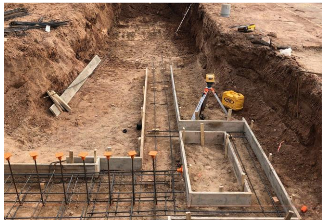
Northwest corner footings being installed.
